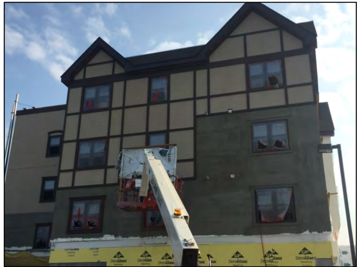
Installation of the Tudor Facade at the Pinebrook Condominiums
