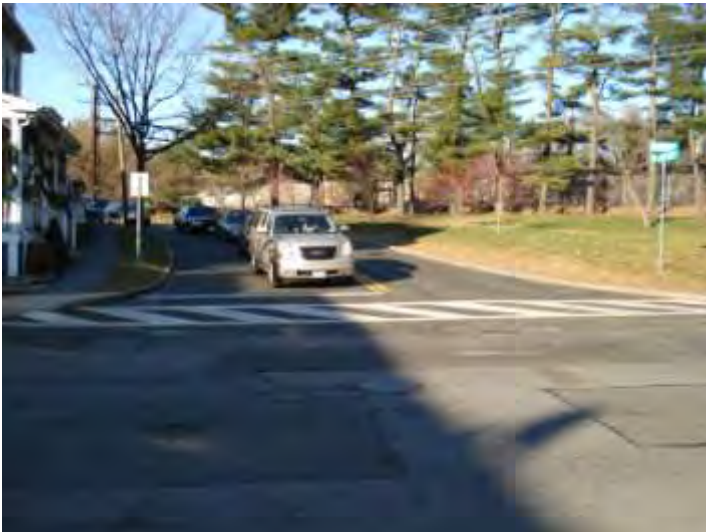
Intersection of Theodore Fremd Avenue & Purchase Street
