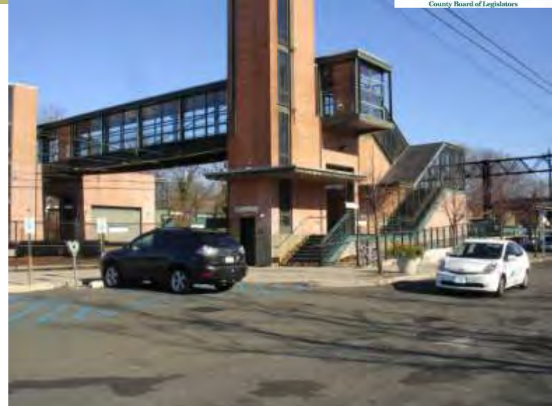
Rye Metro-North Station (above)
