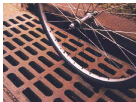
Bicycle-safe drainage grates prevent narrow bicycle wheels from being trapped between grate openings.
