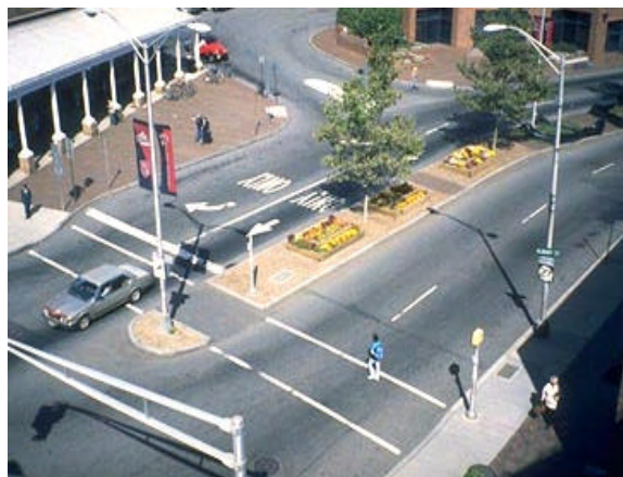
Median islands in the center of the street visually narrow oversized street widths and reduce travel speeds, while also providing a refuge for pedestrians and cyclists in the middle of busy roads.
